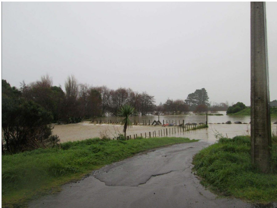
Figure 8: Flooding in Joll Street Reserve (Waitara)
