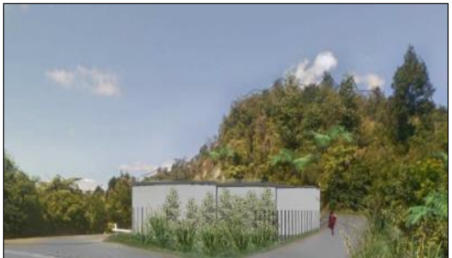
Figure 14: Hydrant Tanks above tunnel
