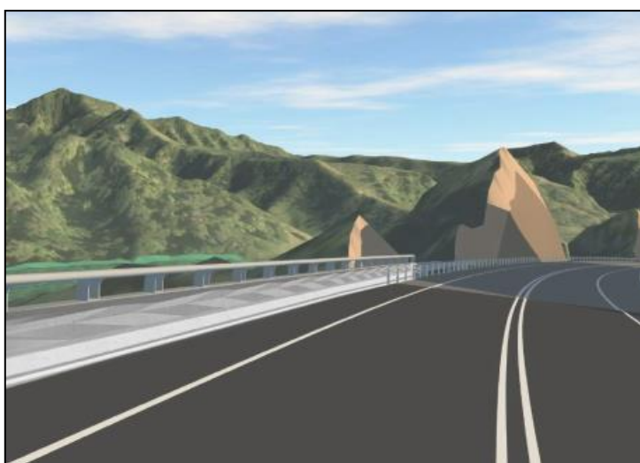
Figure 9: Concrete safety barrier on the bridge
