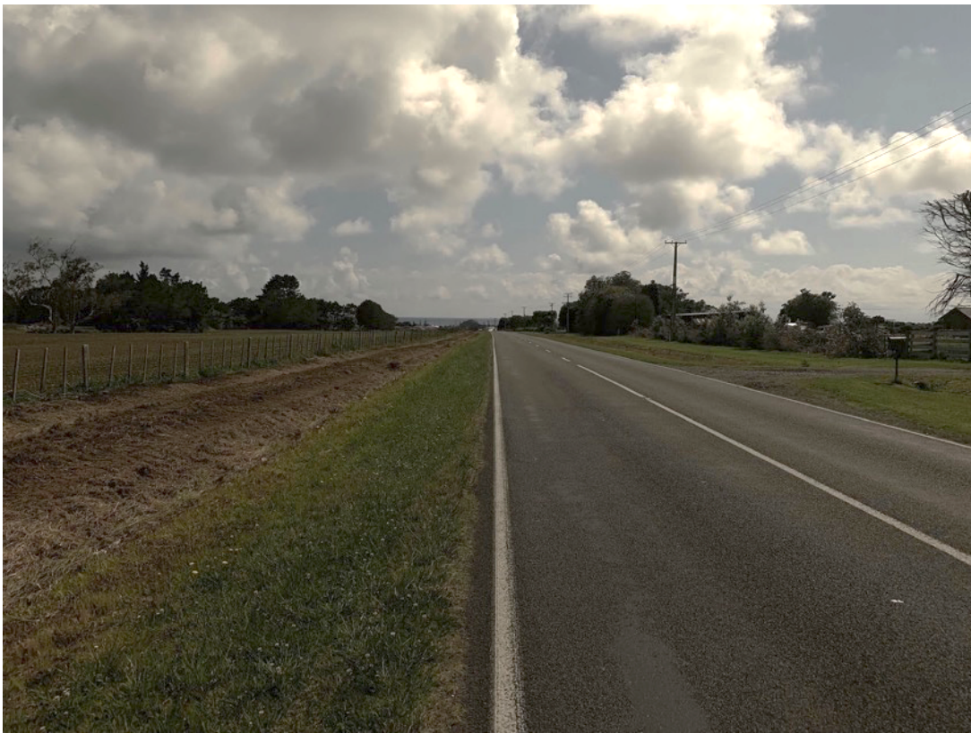
Figure 12. Raleigh Street – looking from Johnston Street Intersection to the North-West
