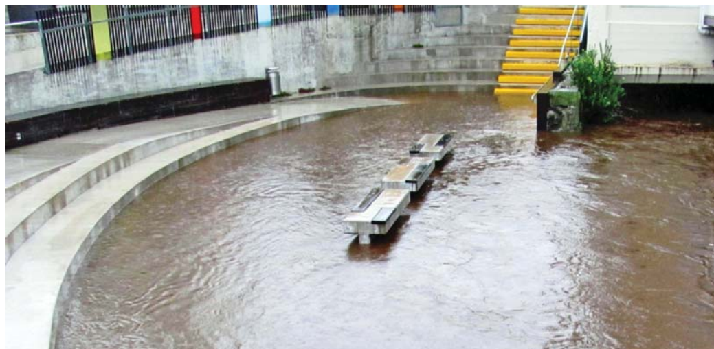
The streamside section of Huatoki Plaza in flood in 2011, as designed, to take the pressure off Huatoki Stream. Do you have a household emergency plan so that everyone knows what to do during floods, earthquakes or other disasters?
