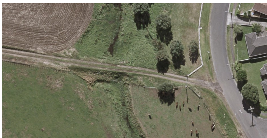
Figure 1. Aerial photo of a recent culvert in the Mangaiti Stream providing access from Ranfurly Street
