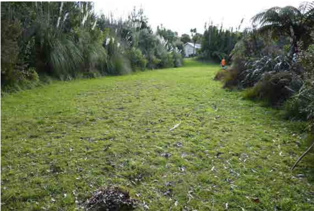
Figure 35: Large bulldozed rear terrace looking north towards the Rowe house. The central rear spur is located on the left and the batter formed by the bulldozing of the terrace is covered in vegetation on the right of the frame.
