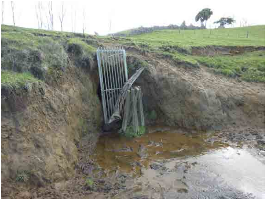
Figure 22: P19/323 Drainage tunnel entrance.
