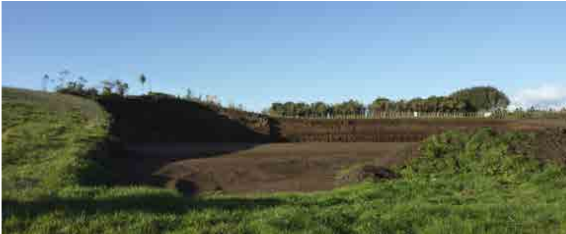
Figure 11: Exposed bank cutting on the boundary of southern boundary of Property 1, facing south towards Property 6.
