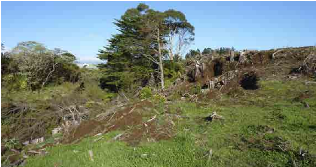
Figure 56: Clearing activity at rear of Property 15.
