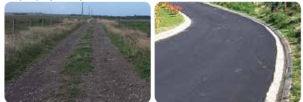
Above: The House for Karen - narrow gravel entrances provide the necessary infrastructure and fit into the rural landscape well.
