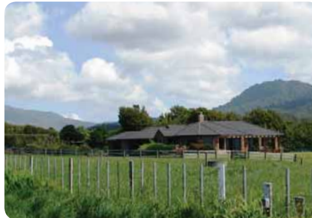
Above: This larger dwelling is accommodated into the rural environment with the use of a detailed hip and gable roof that softens the building's bulk.
