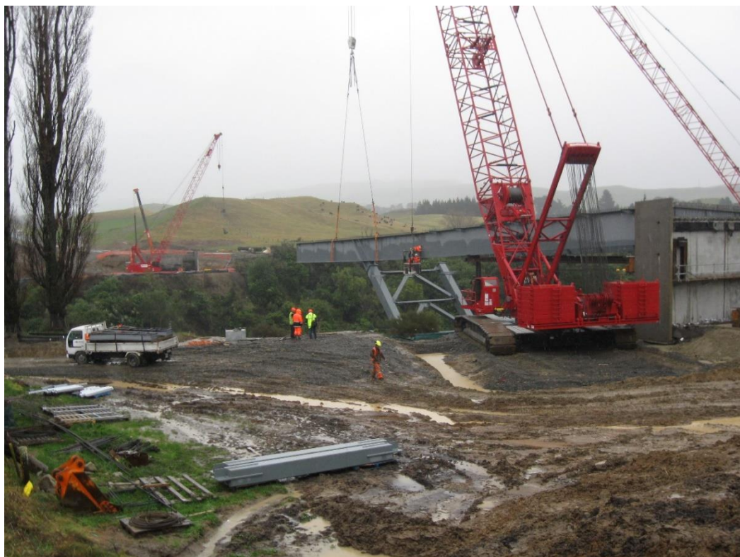
Figure 12: Photograph showing similar size of large crane required for Z option Bridges 1 and 2
