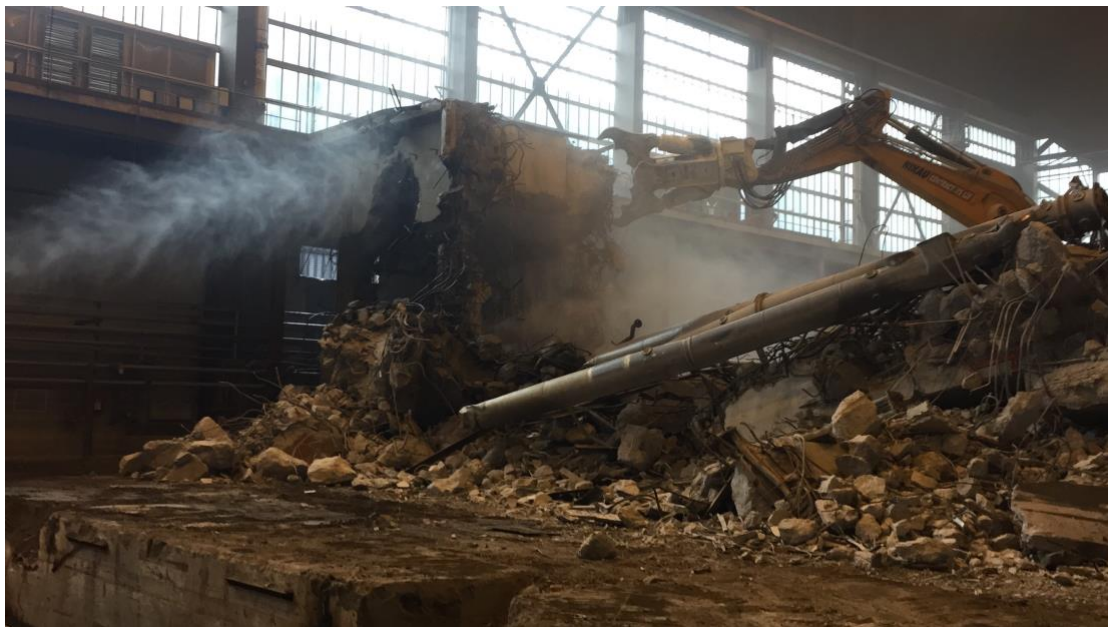
Figure 2 : Atomised water dust and airborne particle suppression
