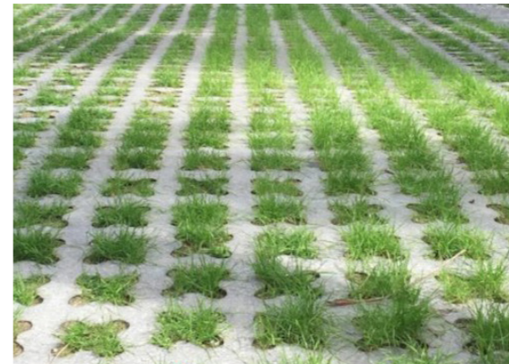
PERMEABLE CARPARK SURFACING
