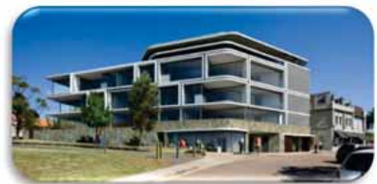
Image 24: Using different forms to help break long linear façade of a building
