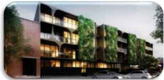
Image 23: Adding interest to the façade with a vertical garden, which also helps to regulate temperature
