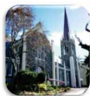
St Mary's Church 1869 Architect: F De J Clere
