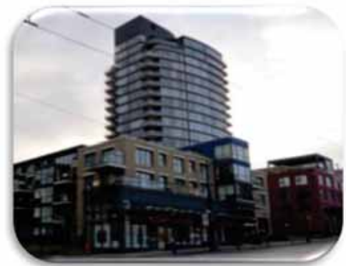
Image 16: Taller building set back from the street edge with low rise buildings in front, in Vancouver
