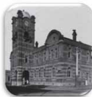
New Plymouth Post Office & Clock Tower 1872 d.1969 Architect: W. H. Clayton
