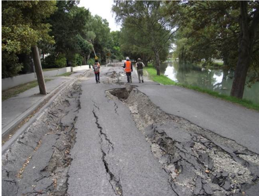
Photo 1 Lateral spreading fissures running parallel to the Avon River in Avonside Drive, Christchurch, February 2011 (Photo D. Beetham, GNS Science).
