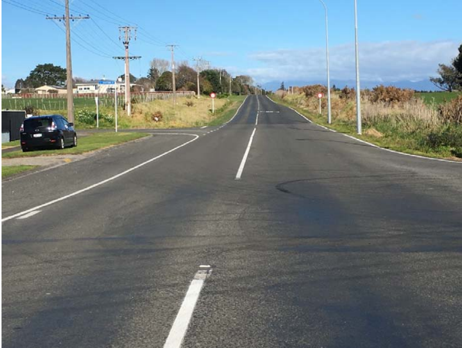
Photograph 1: Raleigh Street – view south from Ranfurly Street intersection
