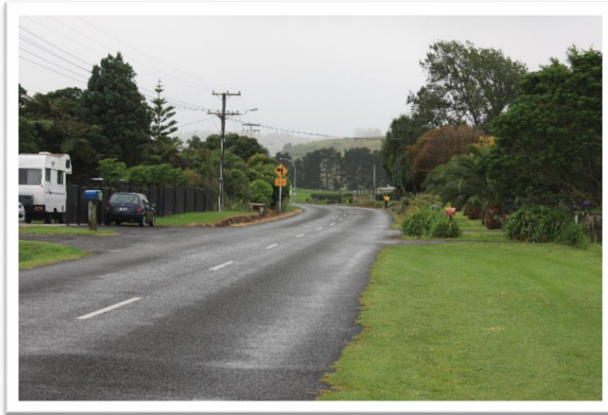
FIGURE 6 - VIEW SOUTH FROM ACCESS
