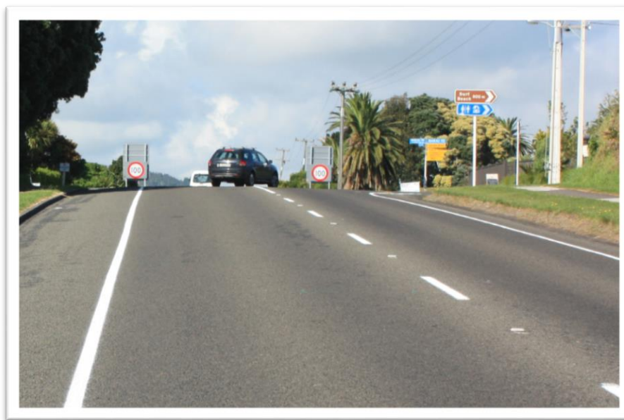
FIGURE 9 - VIEW INTERSECTION FROM EAST
