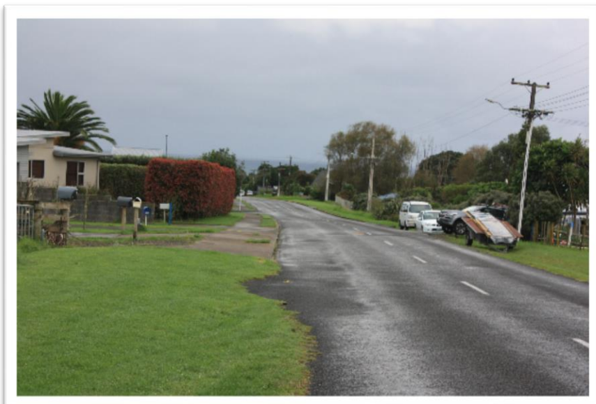
FIGURE 7 - VIEW NORTH FROM ACCESS
