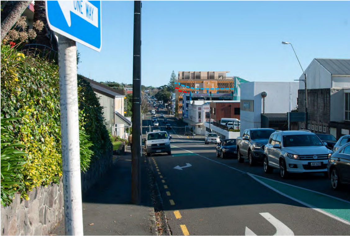
Viewpoint K Simulation – Cnr Liardet & Powderham Streets – Public Receptor (14m ODP approximate building height – (Red dashed line) 17m PDP approximate height (blue dashed line))
