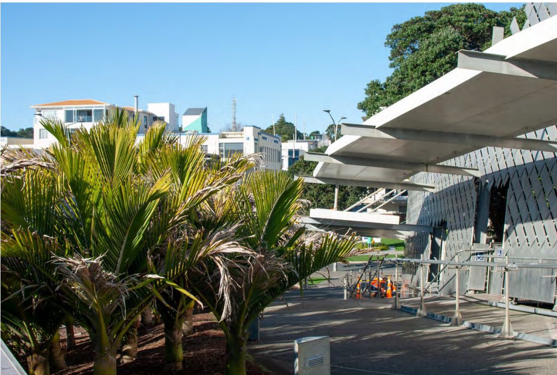
Viewpoint G Existing Condition - Puke Ariki Main Entrance Landing
