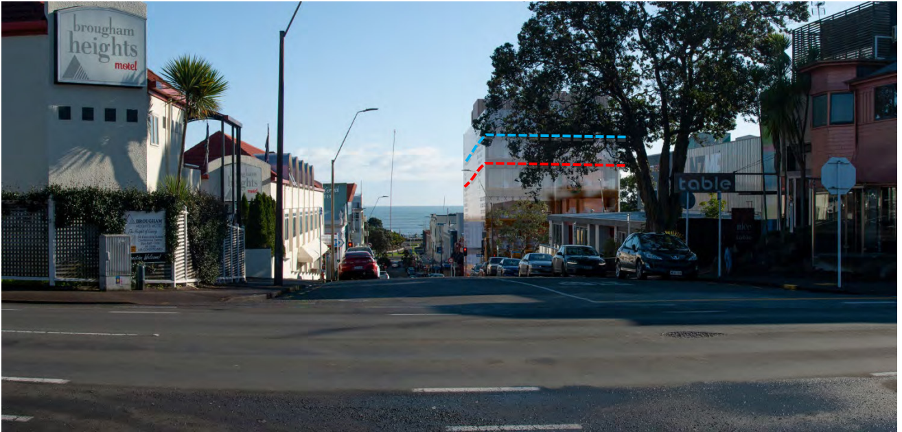
Viewpoint D Simulation – Cnr Vivian and Brougham Streets – Public Receptor (14m ODP approximate building height – (Red dashed line) 17m PDP approximate height (blue dashed line))
