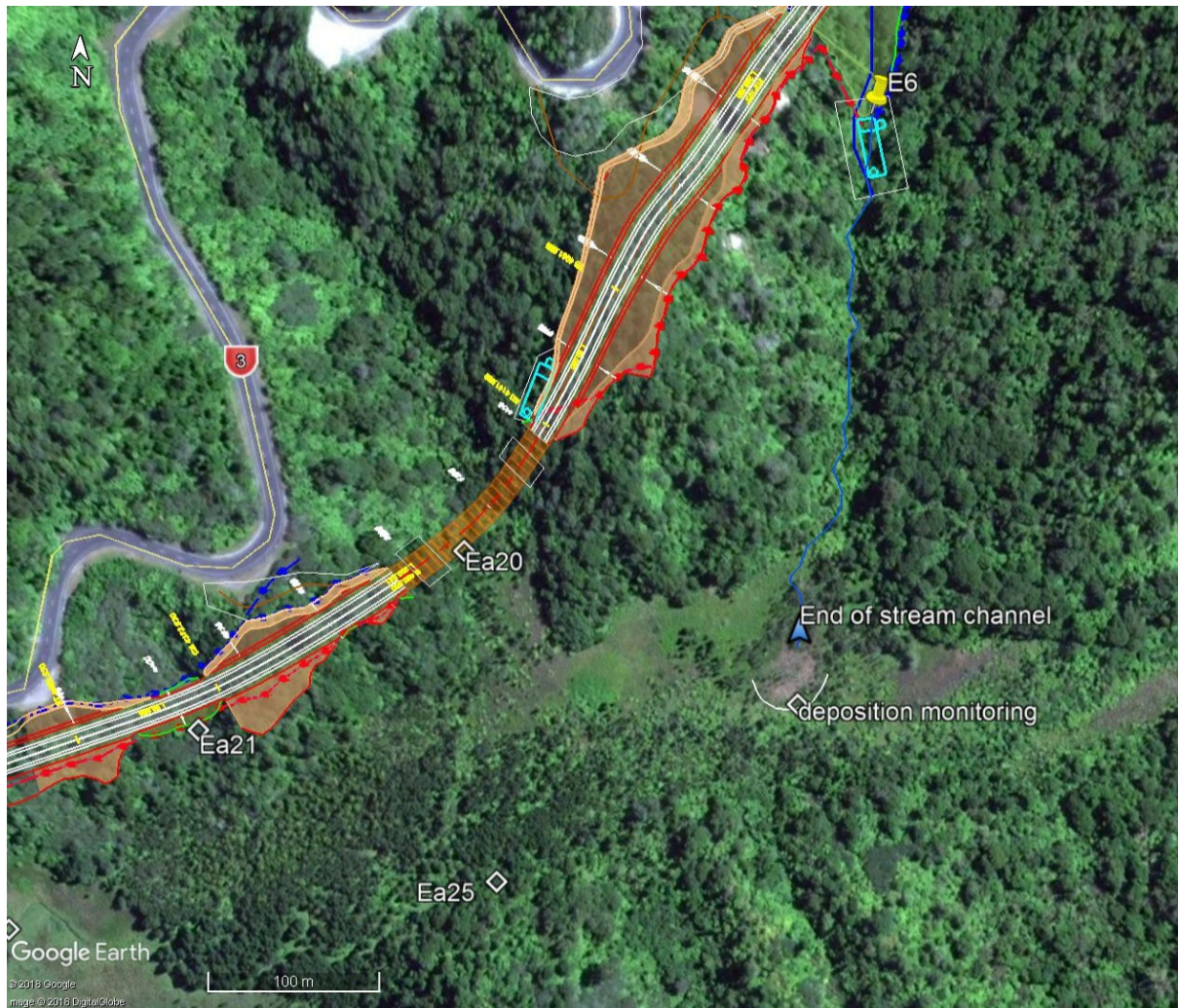
Figure 4.1 – Location of stream channel entering Mimi Wetland and location of sediment deposition monitoring in the event of SRP Management Threshold exceedance
