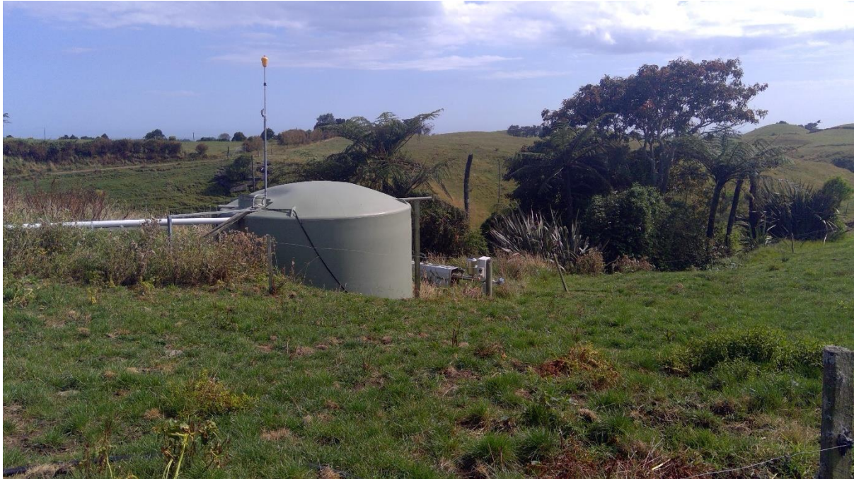
Figure 29: Dairy Shed water tank supplied by bore water and roof runoff. Image 26 February 2021.
