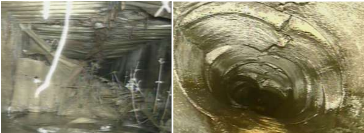
Figure 5.1.4.3 – Failing pipes near Marie Street, Inglewood (left) and under railway near Autere Street (right)
